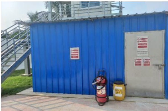
Photo 11: Hazardous Waste Storage Shed
