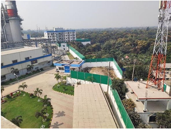
Photo 1: Noise barrier installation on boundary wall
