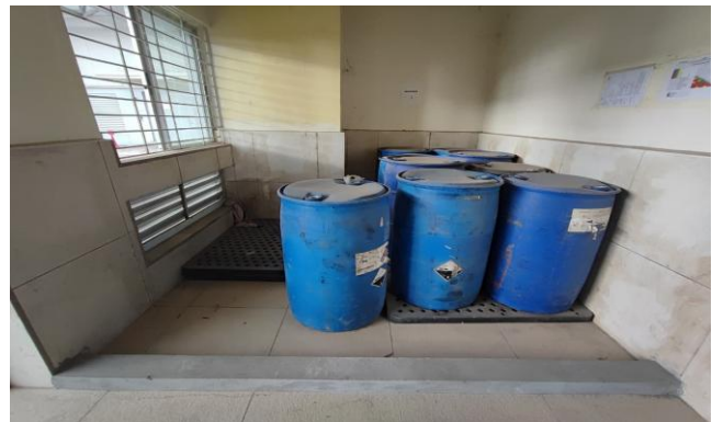
Photo 12: Secondary Containment at Aquas Ammonia Storage Room
