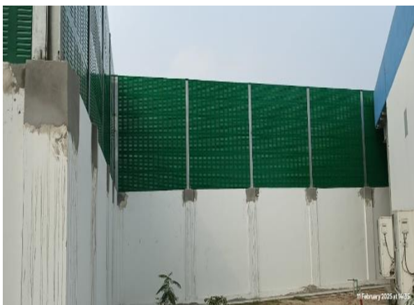
Photo 1: Noise barrier installation on boundary wall
