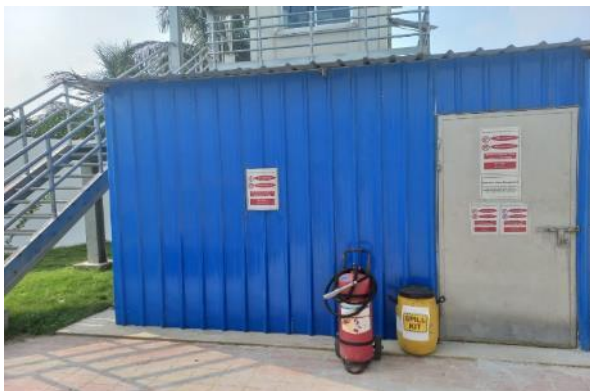
Photo 11: Hazardous Waste Storage Shed
