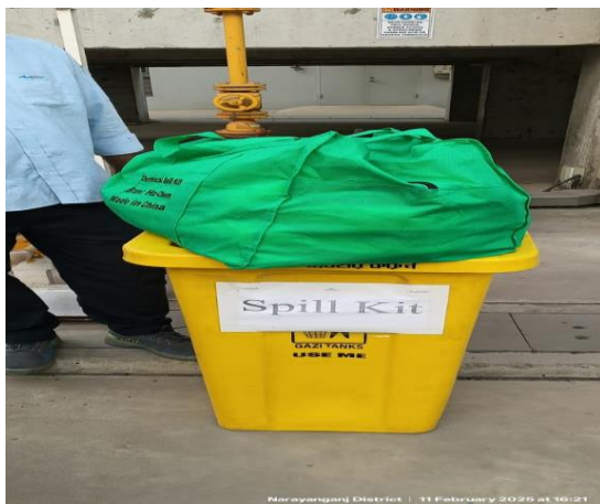
Photo 9: Spill Kit provided near bulk acid-alkali storage
