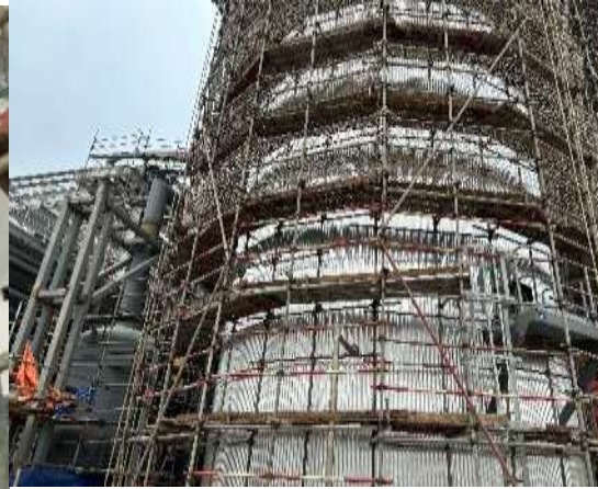
Fig 4: Provision of safety net for exterior height work activities
