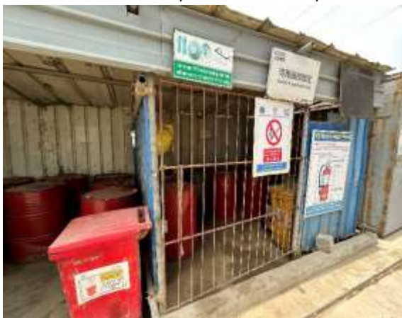
Fig 9: Hazardous waste being storage in designated covered and paved shed
