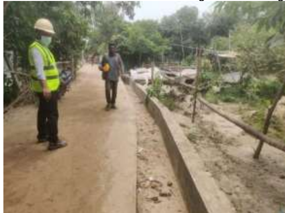
Fig 23: visit to Drainage line construction in Doodhghata village
