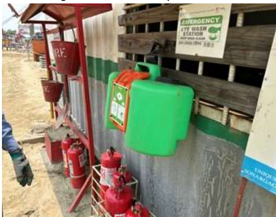
Fig 11: Provision of eyewash station at diesel storage area at construction site
