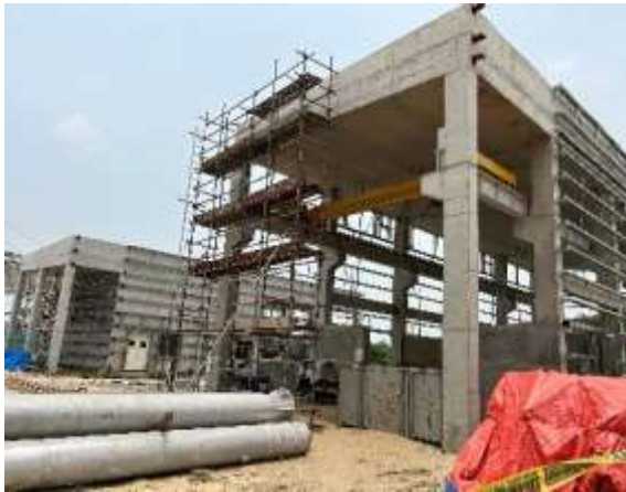
Fig 13: Hydrogenation building under construction onsite
