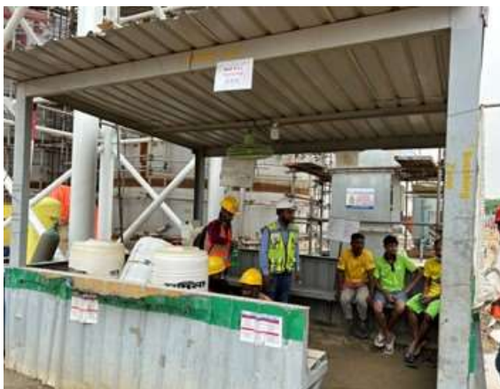
Fig 5: Temporary rest rooms onsite provided with lighting and drinking water centres
