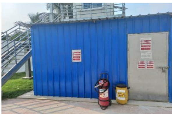
Photo 11: Hazardous Waste Storage Shed
