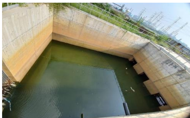
Photo 12: Treated Effluent Storage Basin
