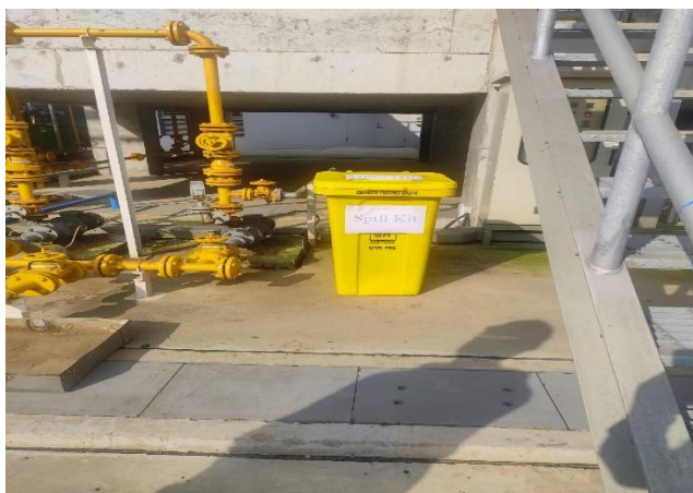
Photo 2: Spill kit provided at acid-alkali bulk storage
