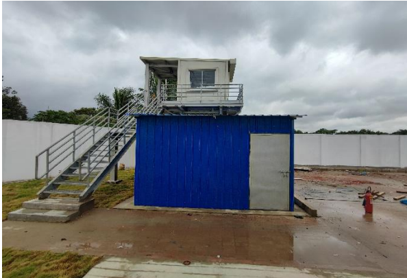
Photo 1: Hazardous Waste storage shed
