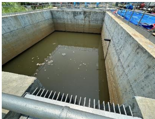
Photo 6: Storm water storage basin
