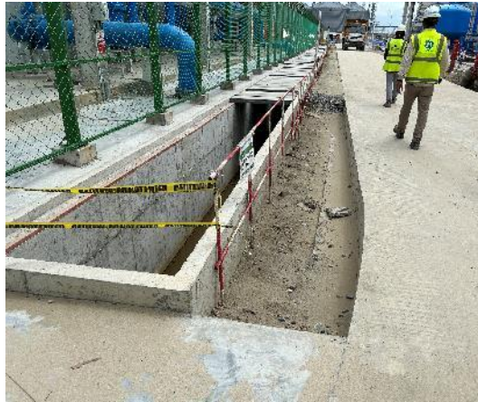
Photo 8: Safe barricading provided at open excavated areas/drains
